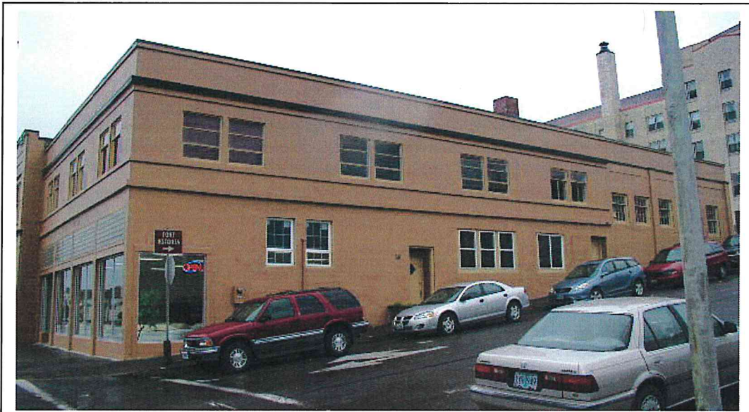
Example: 1511 Commercial – vinyl windows installed years ago that were not paintable. They are white and the building has since been painted brown with brown trimmed windows. The unpaintable vinyl windows remain white and do not blend with the building.
